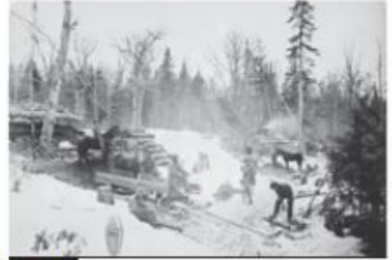
1.67 A logging camp at the end of 19th century where trees were cut to make sawn lumber and firewood. At the time, trees were cut by hand, using a wide variety of axes and saws. The forest industry relied on human and animal power—particularly horsepower.
