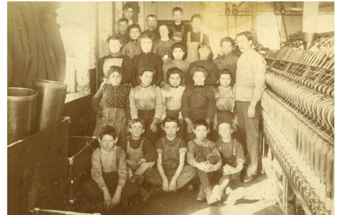
52 Workers in a mill in Montréal, 1891
